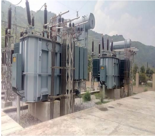
Two Power Transformer Installed
