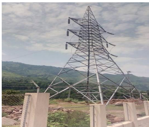
132 KV Incoming transmission line
